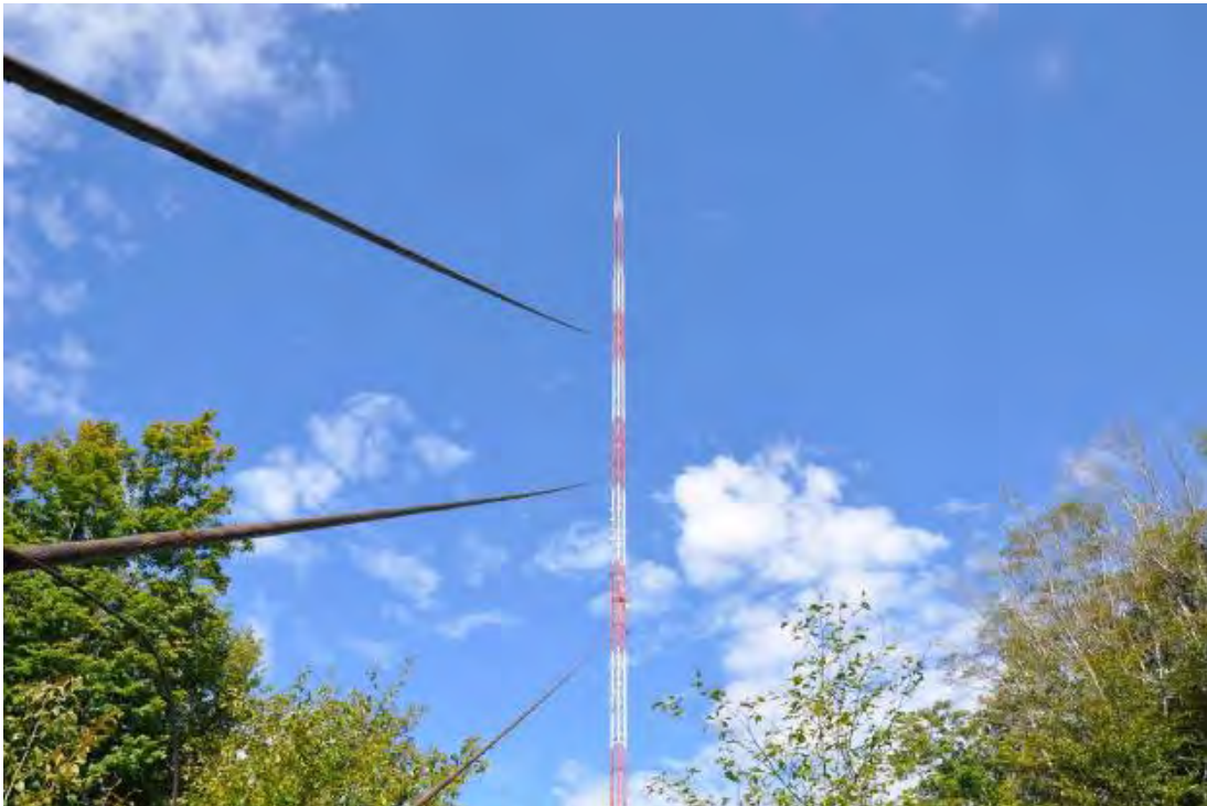
Figure 3. Guy Wires Supporting the WPBN Tower
