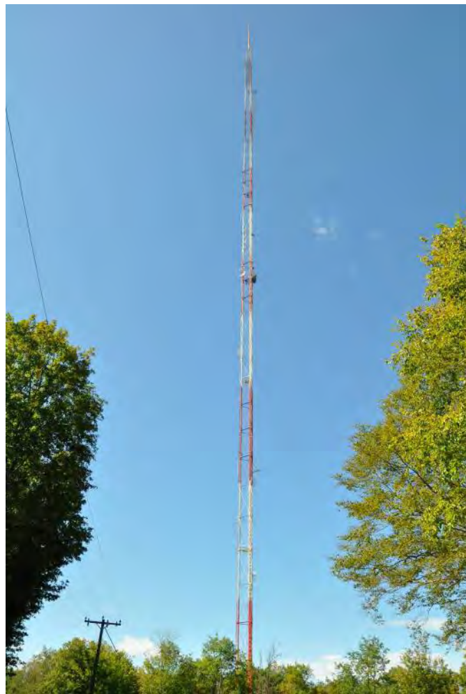
Figure 1. The WPBN Tower, Harrietta, Michigan
